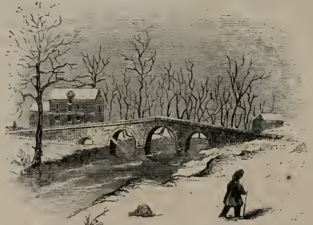
BRIDGE AT WORTH'S MILLS. 3
